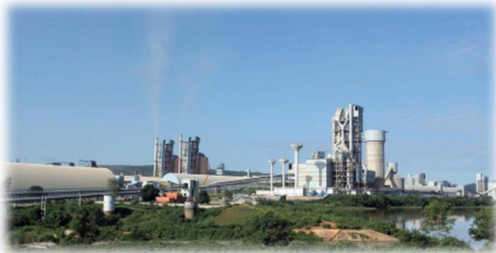
4x6,000t/f Cement Production Line for Dangote Group in Nigeria
