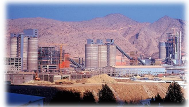
SPCC3x5,000t/d Cement Production Line in Saudi Arabia
